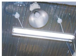
Fluorescent lamp fitted with high-reflectance reflectors
