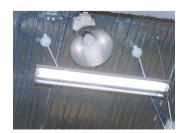
Fluorescent lamp fitted with high-reflectance reflectors
