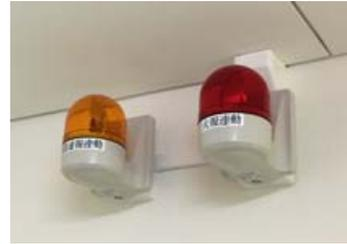
Installation of revolving warning lights in the office and toilets to alert staff of earthquakes, fires, time tone
